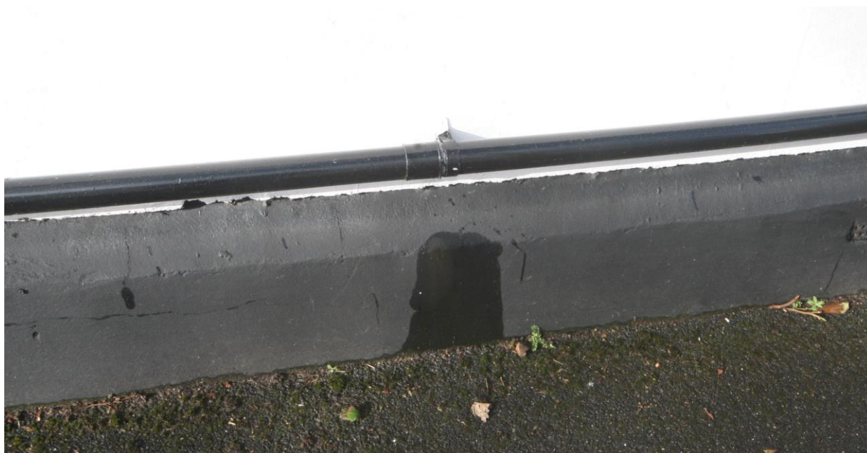
Two dislodged downpipe connections which should be repaired/renewed.
