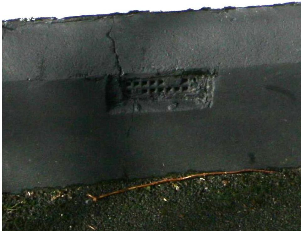
Vents in the plinth should be opened up and maintained
