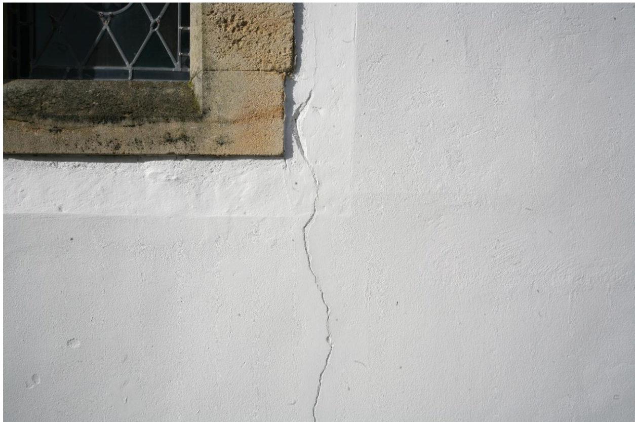
Typical examples of cracks in the cement render – these need filling with silicate filler before the wall is painted with the silicate paint system.
