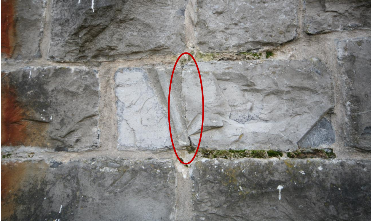
An example of a joint opening up which can allow moisture ingress even if the crack is only hairline. This should be raked out and repaired in lime mortar.
