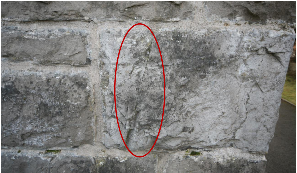
Small hairline fissures in the stones can potentially draw moisture through
